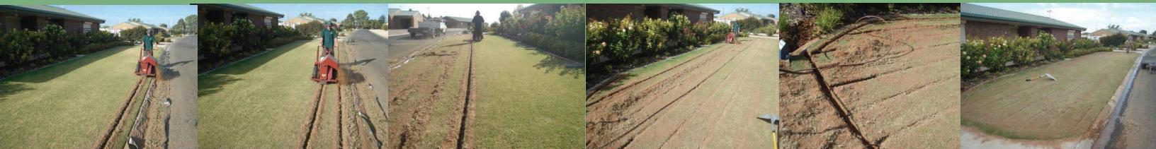
**SDI step by step installation using the TRENCH'N edge Trencher.**
