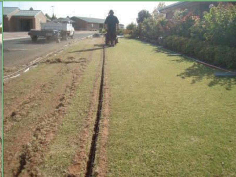
**Continue blowing the trenched material directly into each of the previous holes after you install the SDI line.**
