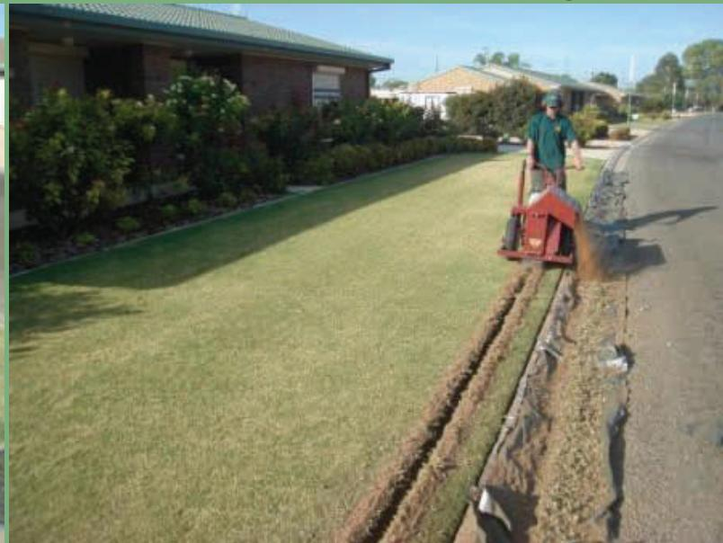
**First trench – blow onto tarps and hold trench material for use filling the final trench.**
