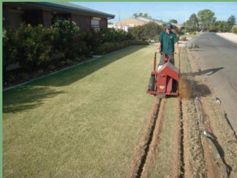
**Second Trench – Blow the trenched material directly into the first trench, after you have installed the SDI line.**
